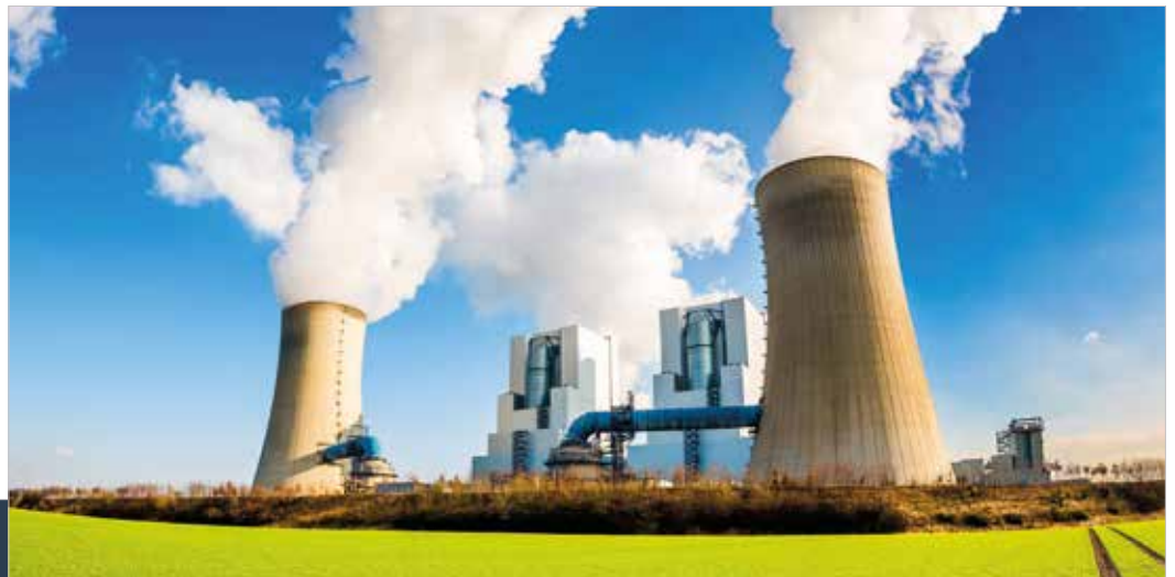
Power stations and incineration units
